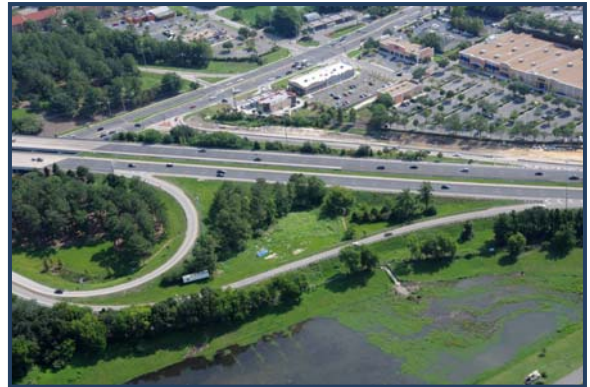
Aerial photo showing the I-75 at SR 26 Ramp
