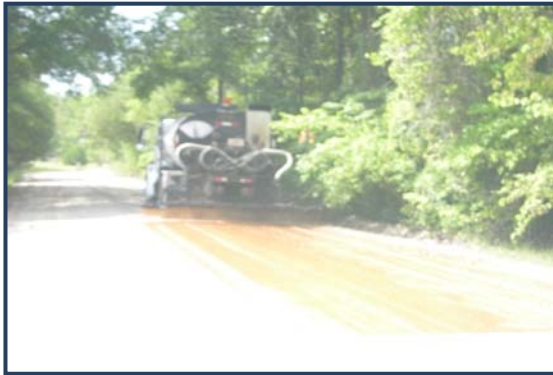
Photo of Lignin LS-50 being applied
